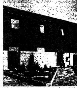
Simber Research Limited at Merthyr Tydfil was winner of category 1, with a timber frame, highly insulated two-stoney building Storage fan heaters, panel convectors with close tolerance thermostats plus limited air conditioning maintain prescribed conditions for clinical drug trials.
